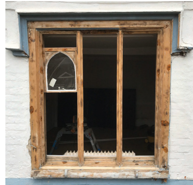
Left: Triple, lancet head unit stripped prior to repairs
